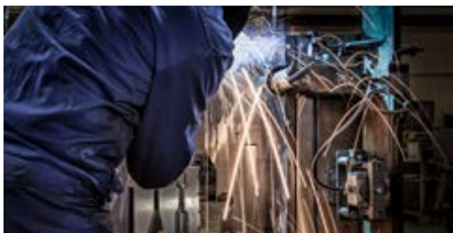
Welding of frame
